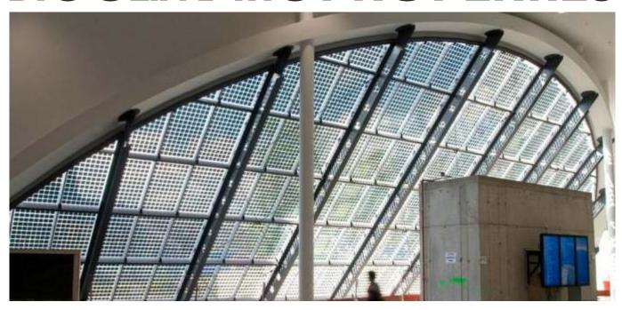
In addition to an undeniable aesthetic value, these are solutions that combine active properties (photovoltaic generation) with passive properties such as thermal and acoustic insulation, natural lighting and selective filtering of the harmful components of solar radiation.
